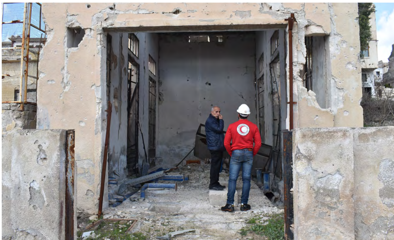
Rehabilitation of the Handrat water supply center in Syria. Image credit ICRC.
